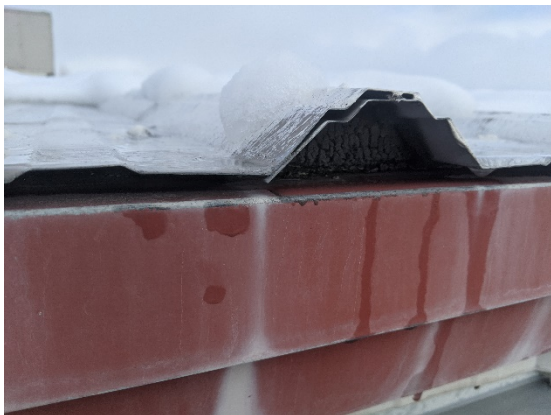
Roof edge and flashing
