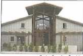
The exterior style of the Lake Chelan has been approved. Seven Acres Foundation's prime contractor, Rimmer and Roeter, is currently discussing design and structural constructability with Butler Manufacturing, specifically on the mechanical. Get involved. We are continuing forward.
