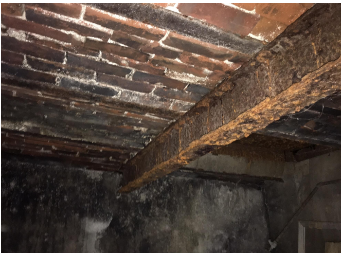
5. Framing Under Sidewalk
