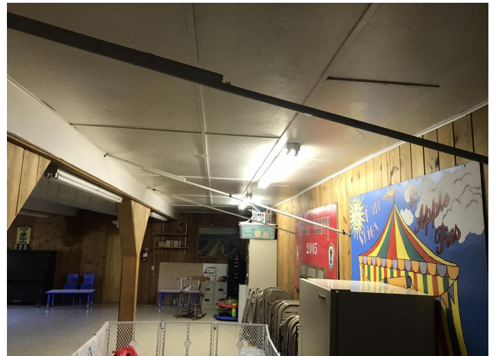
6. Tie-backs in Bottom/Lower Floor
