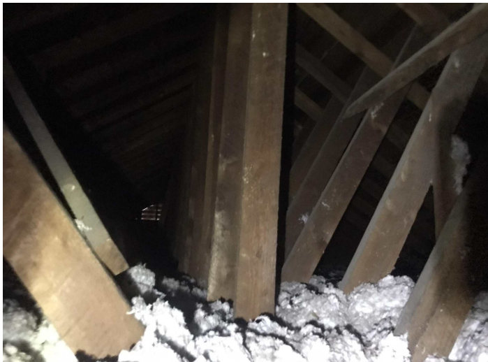
3. Existing Roof Trusses
